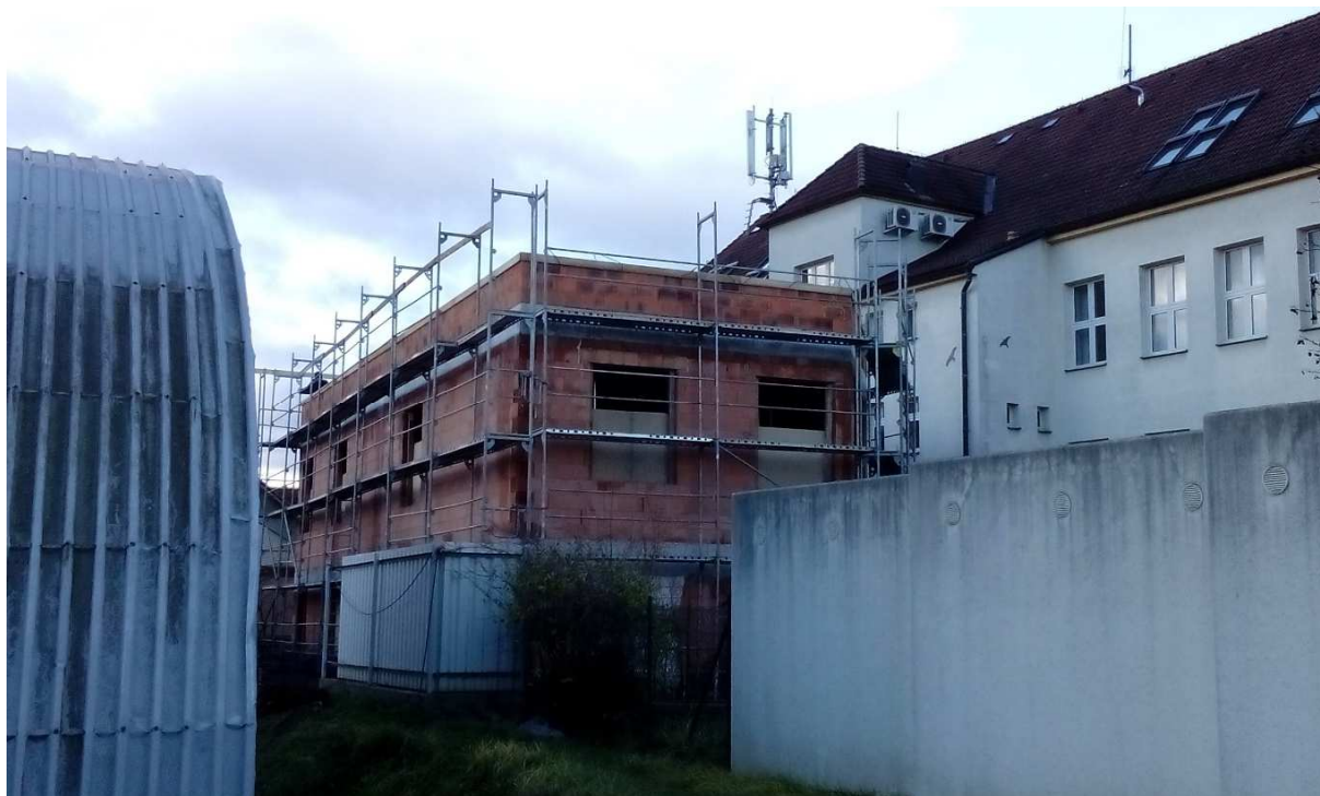
Course of construction works at the SLNO building. Photo: USB archive.
